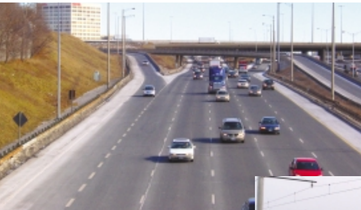
Figure 1 As they merge onto the main expressway lanes, cars and motorcycles accelerate more easily than trucks.
