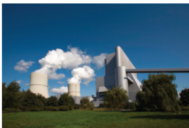
Figure 1 This coal power plant in Spremberg, Germany, uses carbon capture and storage.
